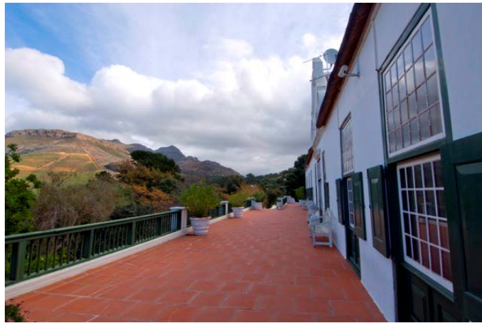
Front Exterior View
